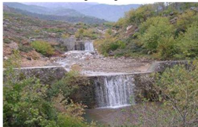
Fig No. 8 Embankment built with concrete
